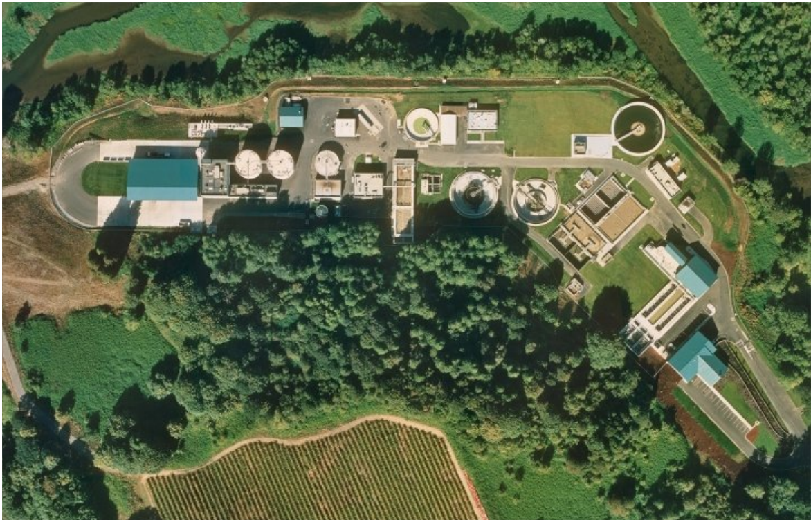
Figure 2. Salmon Creek WWTP in Clark County, Washington.
